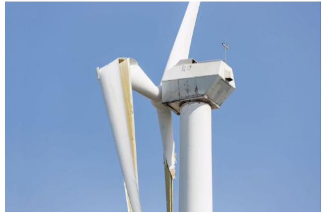
Figure 1b: Lightning damage to a wind turbine
