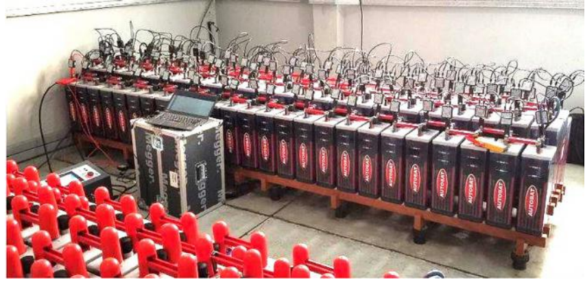
Figure 4: Discharge test setup with BVMs for cell voltage measurement
