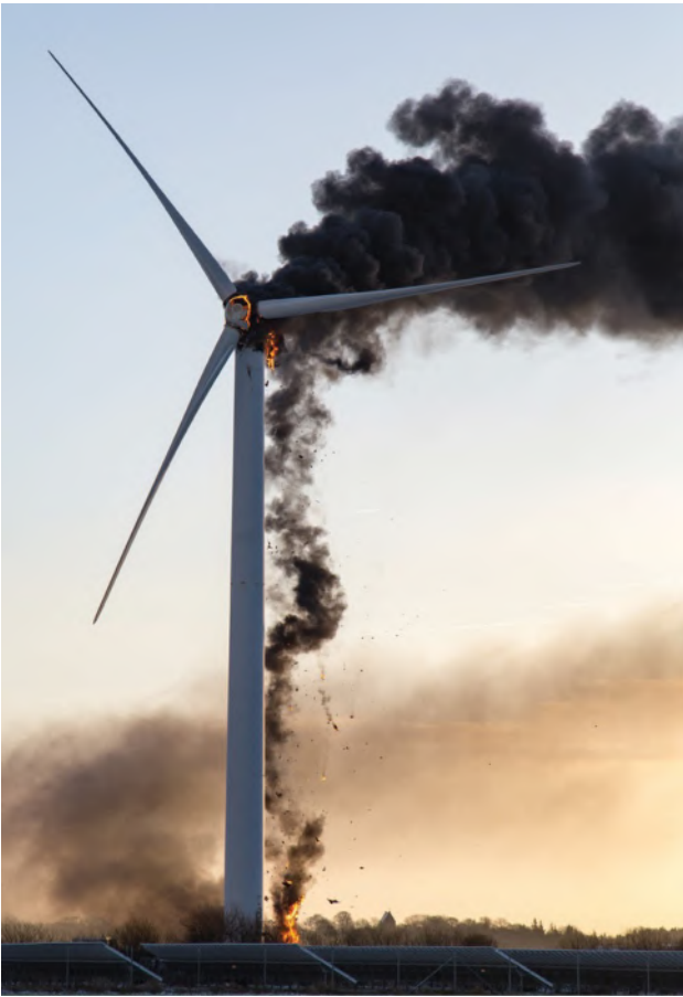
Figure 1a: Lightning damage to a wind turbine
